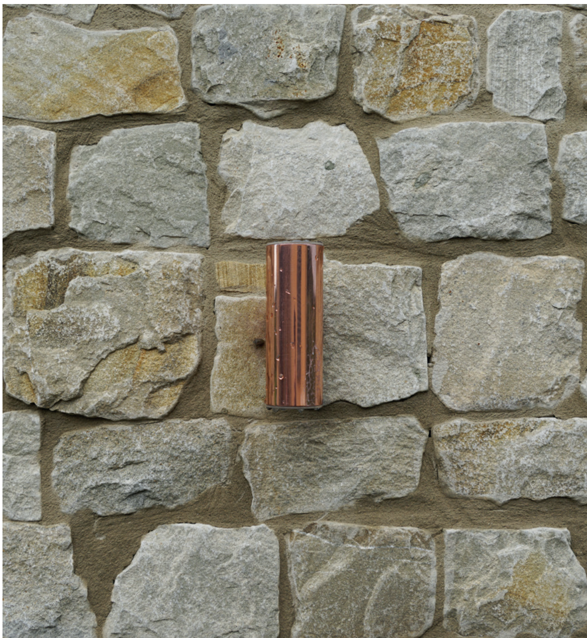
Residenza privata, Scarperia (FI) Private house, Scarperia (FI)
